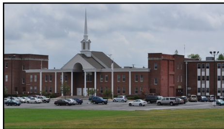
The new home of Tall Oaks Classical School!
